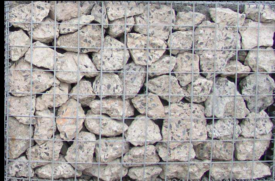
RECYCLED CONCRETE IN GABIONS
