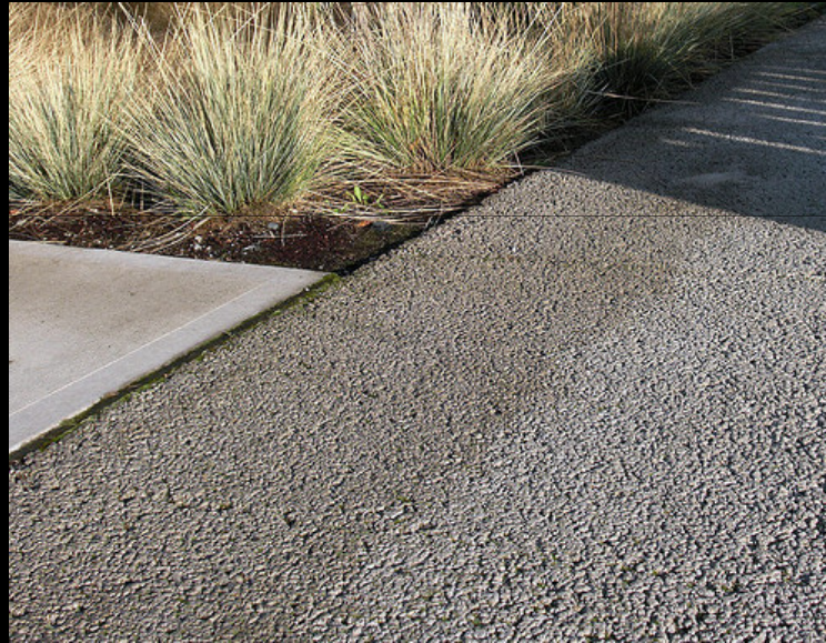
POROUS CONCRETE PAVING
