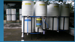
4,000 Liters IRHS Installation : Apostolic Catholic Church, 1003 EDSA, Q.C.
