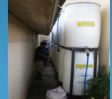
4,000 Liters IRHS Installation: HANBI ICT Center, Navotas City
