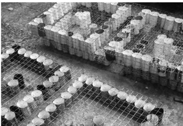
Fig. 12 A cross-section of the panel shows the cardboard core assembly reinforced by wire mesh
