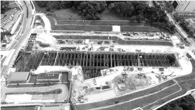
Fig. 10. Bird-eye view of cut and cover tunnel excavation
