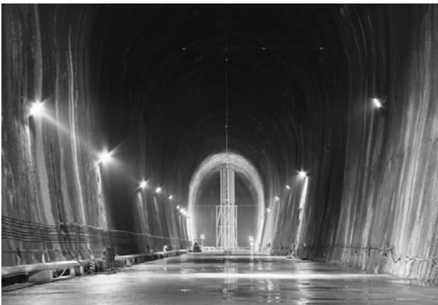
Fig. 2. Underground LPG storage (Japan Oil, Gas and Metal National Corp et al., 2014)
