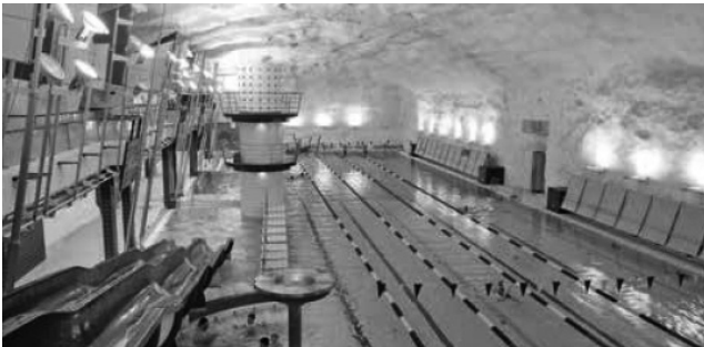
Fig. 1. Underground swim pool in Helsinki (City of Helsinki, 2014)
